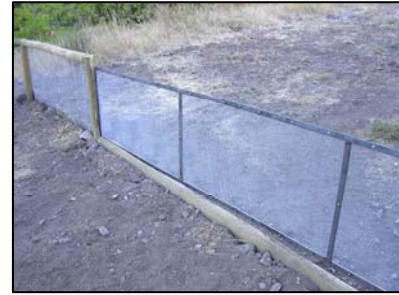
A gate fashioned from mesh and metal frame that slides into channels cut into the posts and a bottom rail.
